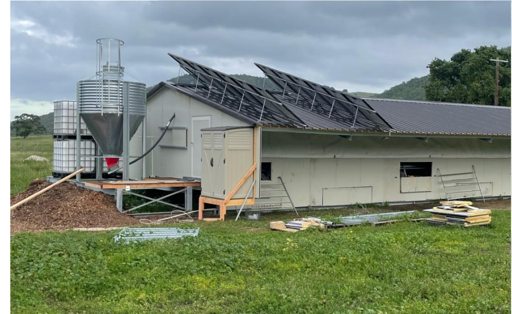
Above: Solar Panel Reuse Project for Chicken Coop. 4/2026 – Marin County.
