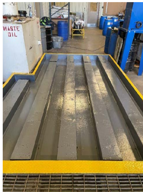
The Marin HHW Facility after its quarterly maintenance and cleaning.
