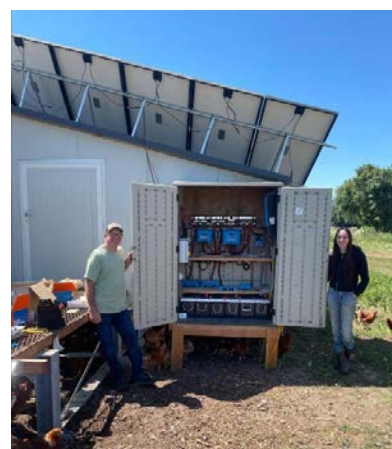
A chicken coop received repurposed solar panels to electrify the building.
